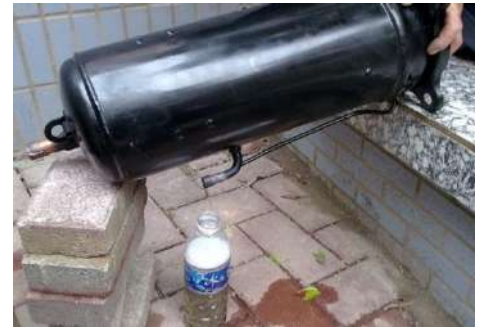
Figure 6-2.8: Draining oil from a compressor
