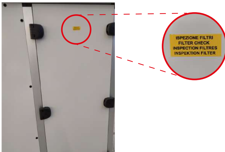
Fig. 24 Panel giving access to filters
