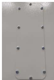
Fig. 8 Blind flange for the connection to the power supply (view from the bottom of the electrical cabinet)
