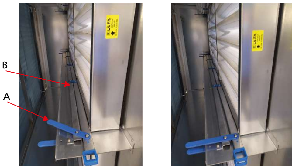
Fig. 25 Filter locking system
