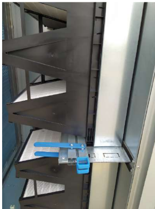
Fig. 27 Modification with filters in place
