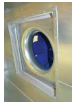
M0 fire class fan flexible connection
