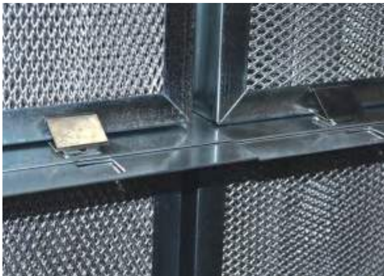
Tightening clip for front withdrawable filter
