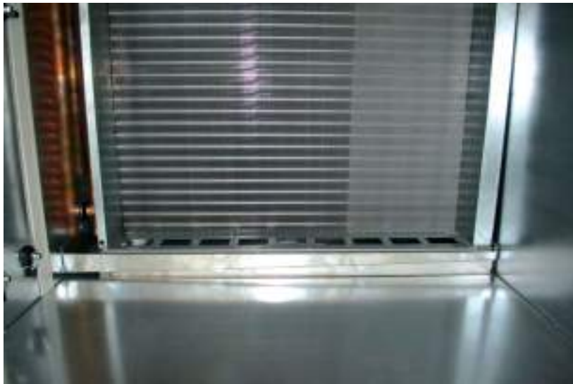
Sloped drain pan
