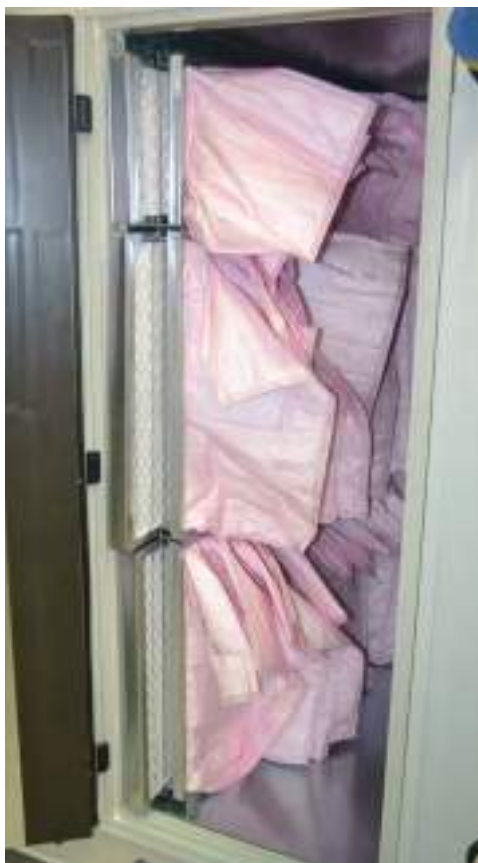
Side withdrawable combined filter (panel + bag)
